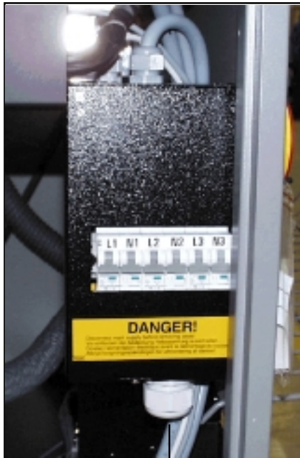
Fig. 3-L Feed power cable through
